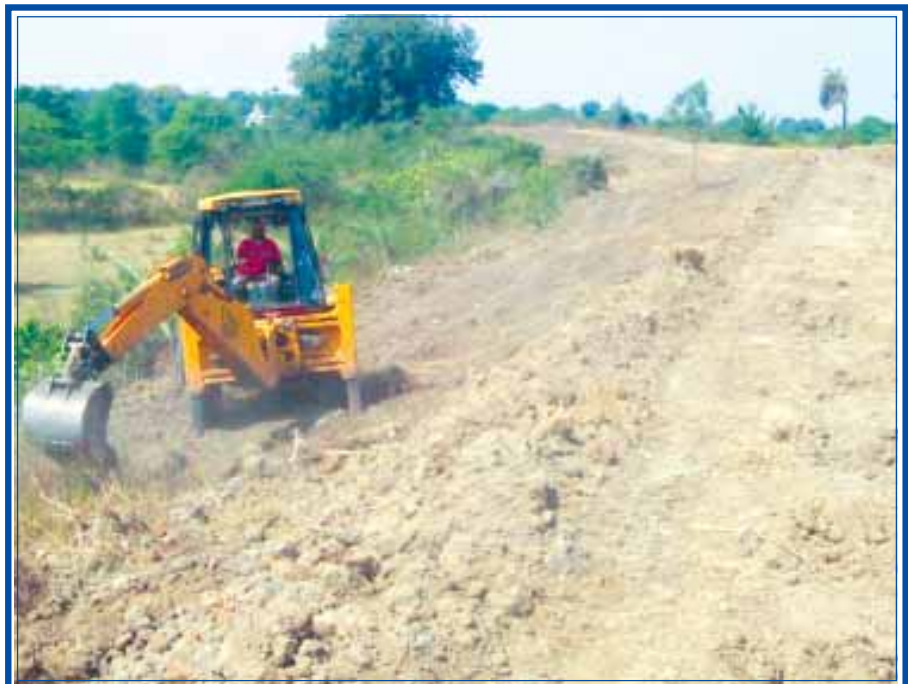
FIG: 1 JUNGLE CLEARANCE IN PROGRESS
