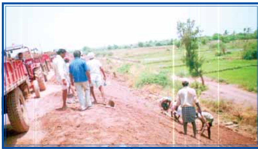
FIG: 7 TRIMMING OF D/S SLOPE - IN PROGRESS
