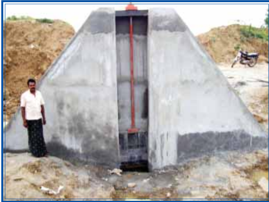
FIG: 8 RE-CONSTRUCTED SLUICE GATE WITH SCREW ROD & GATE
