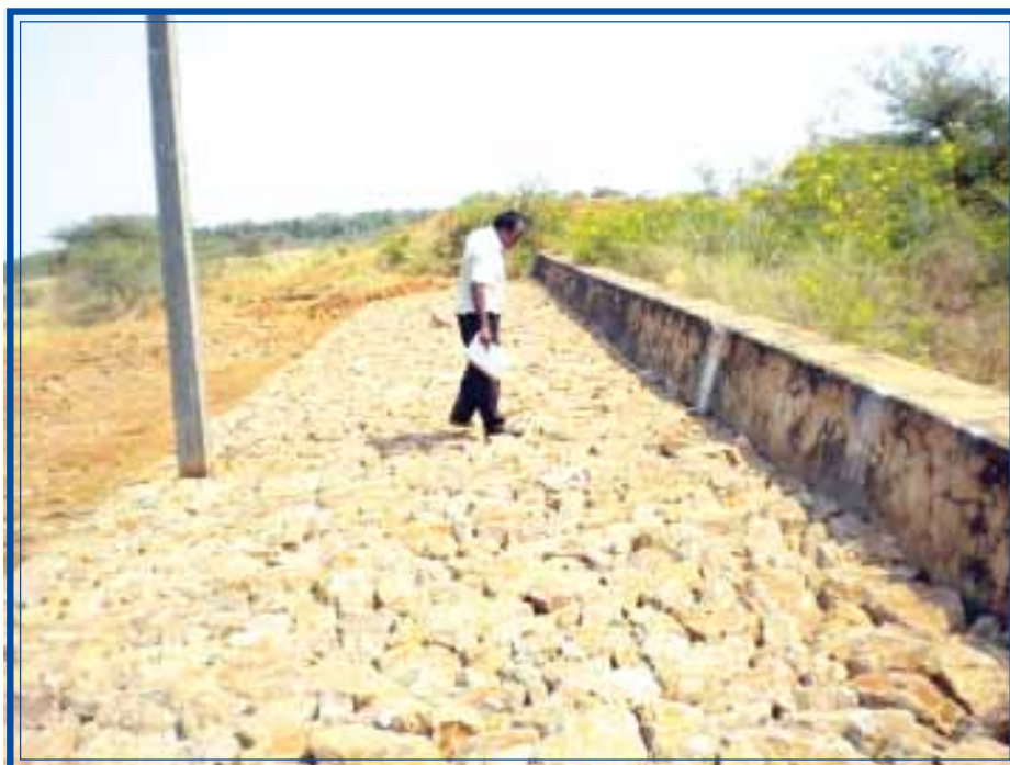
FIG: 14 TALUS -WORK COMPLETED ON D/S OF WEIR
