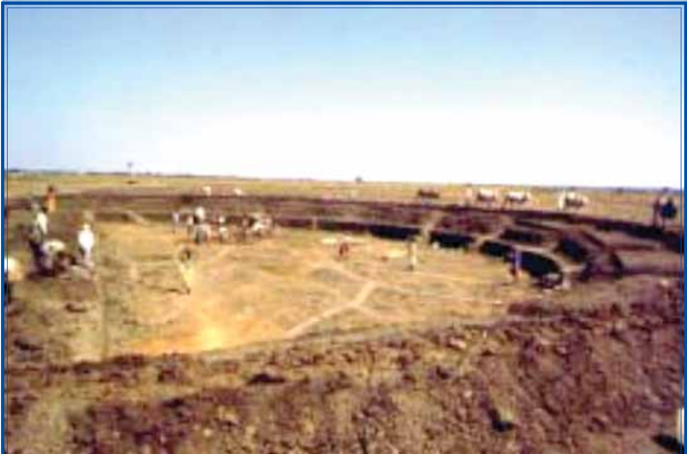
The Dry bed of a small water harvesting structure being cleared.
