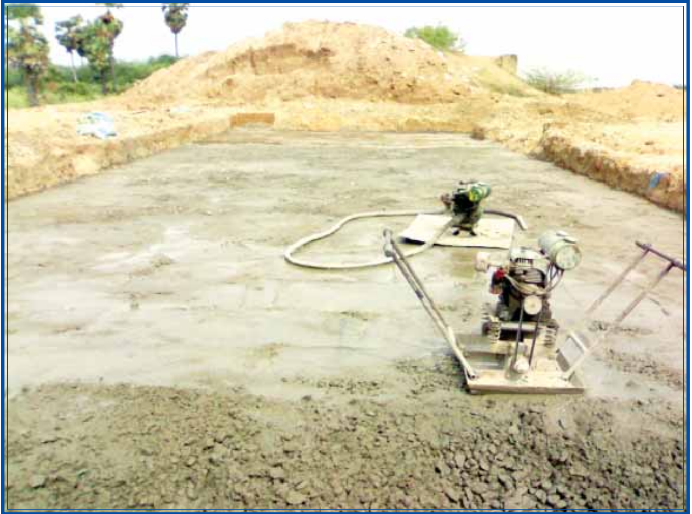
FIG:22 COMPACTION OF CEMENT CONCRETE USING VIBRATORS
