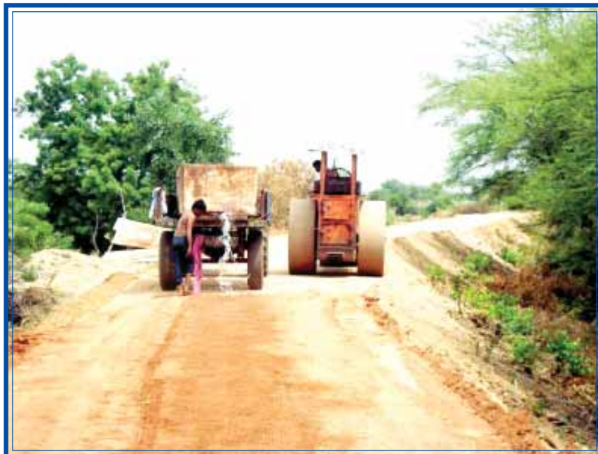
FIG: 3 UNDESIRABLE METHOD OF MOISTENING THE BUND ADVISABLE TO USE GARDNER CAN OR SPRINKLER HOSE ATTACHED
