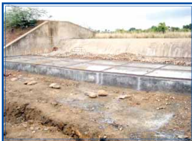
FIG: 11 RE-CONSTRUCTION OF APRON COMPLETED AND REPAIRS TO BODY WALL TO BE TAKEN UP
