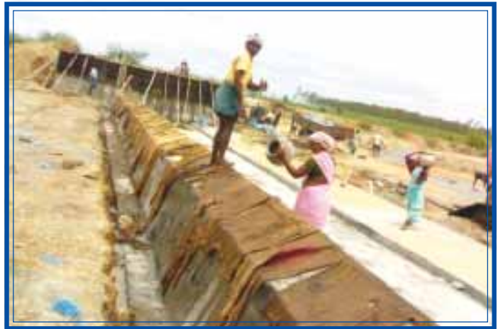
FIG: 13 REPAIRS TO SURPLUS WEIR IN PROGRESS
