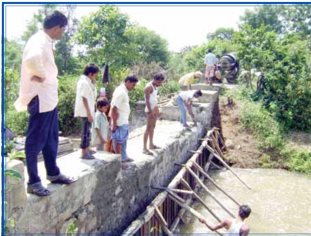
FIG: 16 CLADDING CONCRETE
