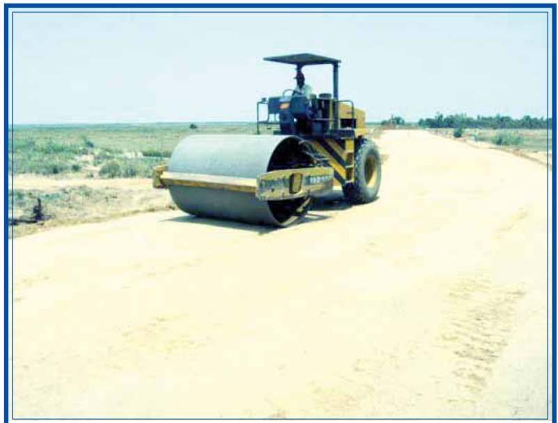
FIG:4 COMPACTION WITH VIBRO MAX ROLLER
