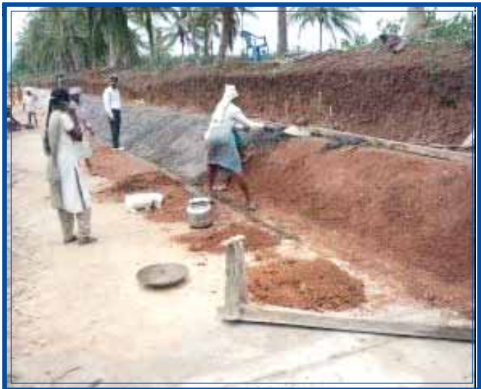
FIG: 17 MANUAL LINING - IN PROGRESS
