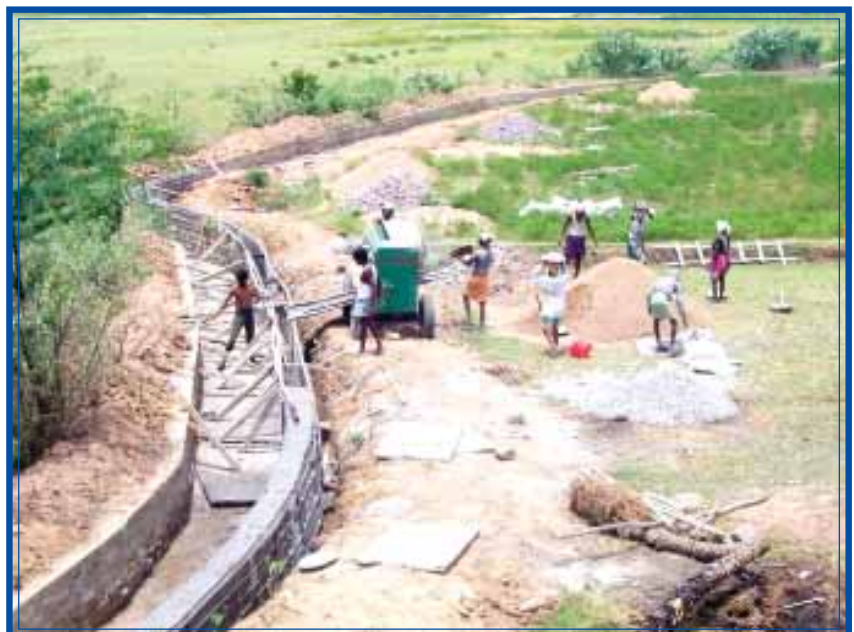
FIG: 20 GUIDE WALL UNDER CONSTRUCTION WITH CEMENT CONCRETE
