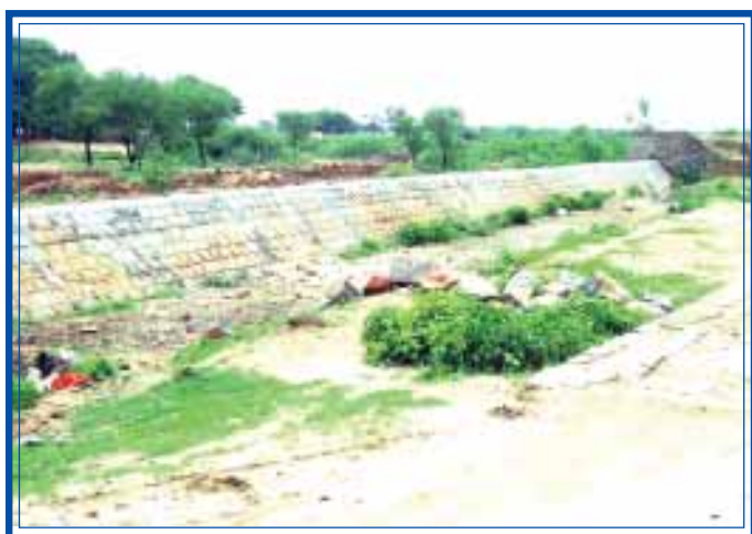
FIG:10 POINTING TO JOINTS IN THE MASONRY WEIR
